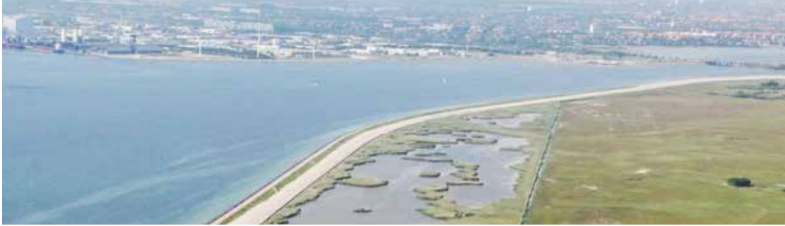
Figure 2 Copenhagen's coastal protection solution – constructing a new dike behind an older dike to protect infrastructure and nature whilst providing a coastal path for recreation (Image: Danish Nature Agency/Martin Nielsen sourced from the Confederation of Danish Industry)
